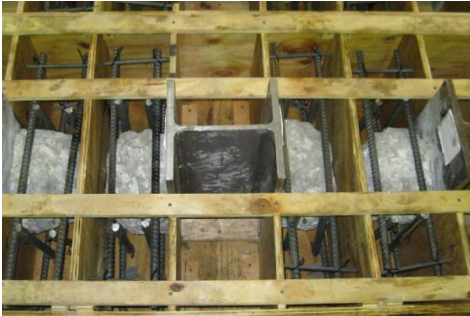
Figure 43. A photograph of specimens, reinforcing steel, and formwork (Dang 2013)
