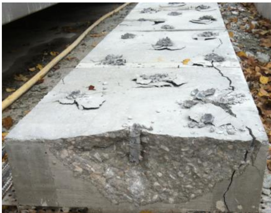
Figure 36. A photograph of chemical splitting on day six (Dang 2013)
