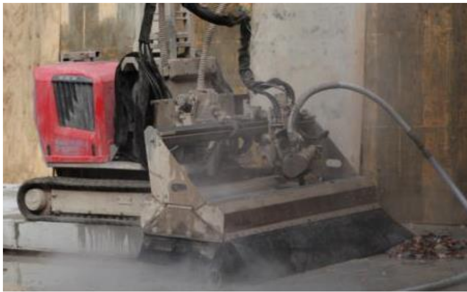
Figure 9. A photograph of the hydrodemolition trial (Dang 2013)
