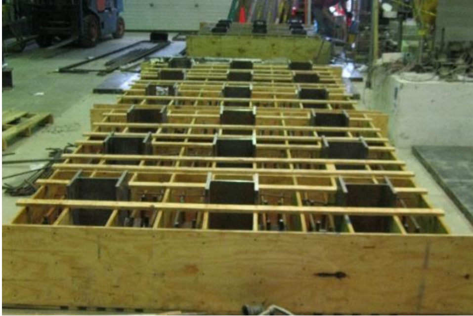
Figure 42. A photograph of partially removed concrete specimens and formwork (Dang 2013)
